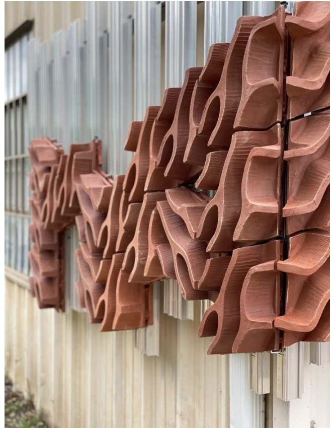
Figure 3. Terracotta as a facade cladding has seen a resurgence in the 21st Century. Shown above is a concept for a self-shading terracotta facade system supportive to local wildlife with nesting areas, produced using digital tooling and ram press technologies. Image credit: Author's design-build studio project.
