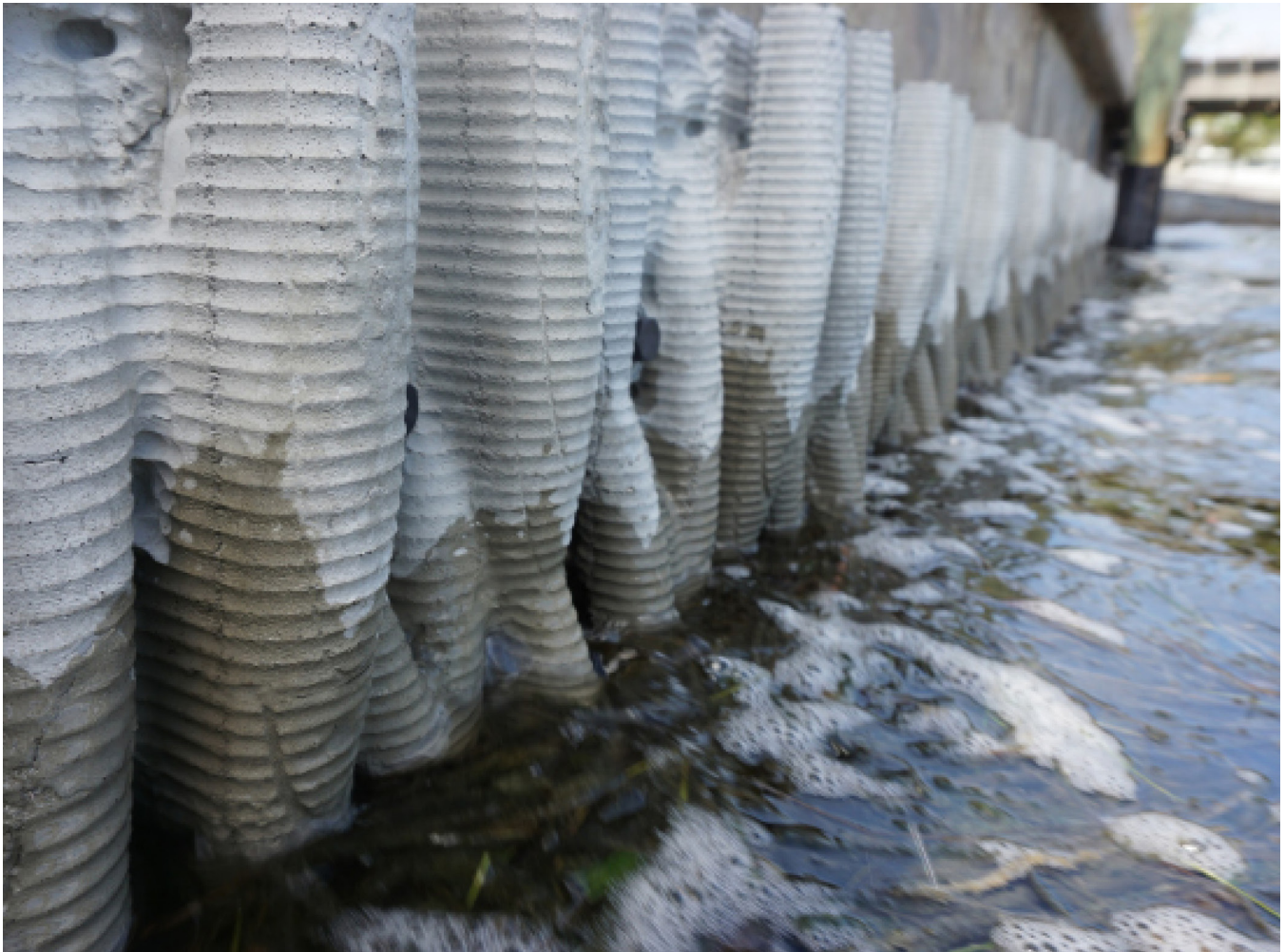
Figure 9. Detail view of texture on prototype panels installed in Southwest Florida. Marine-friendly concrete was used to accelerate recruitment of marine life. Image credit: Author.
